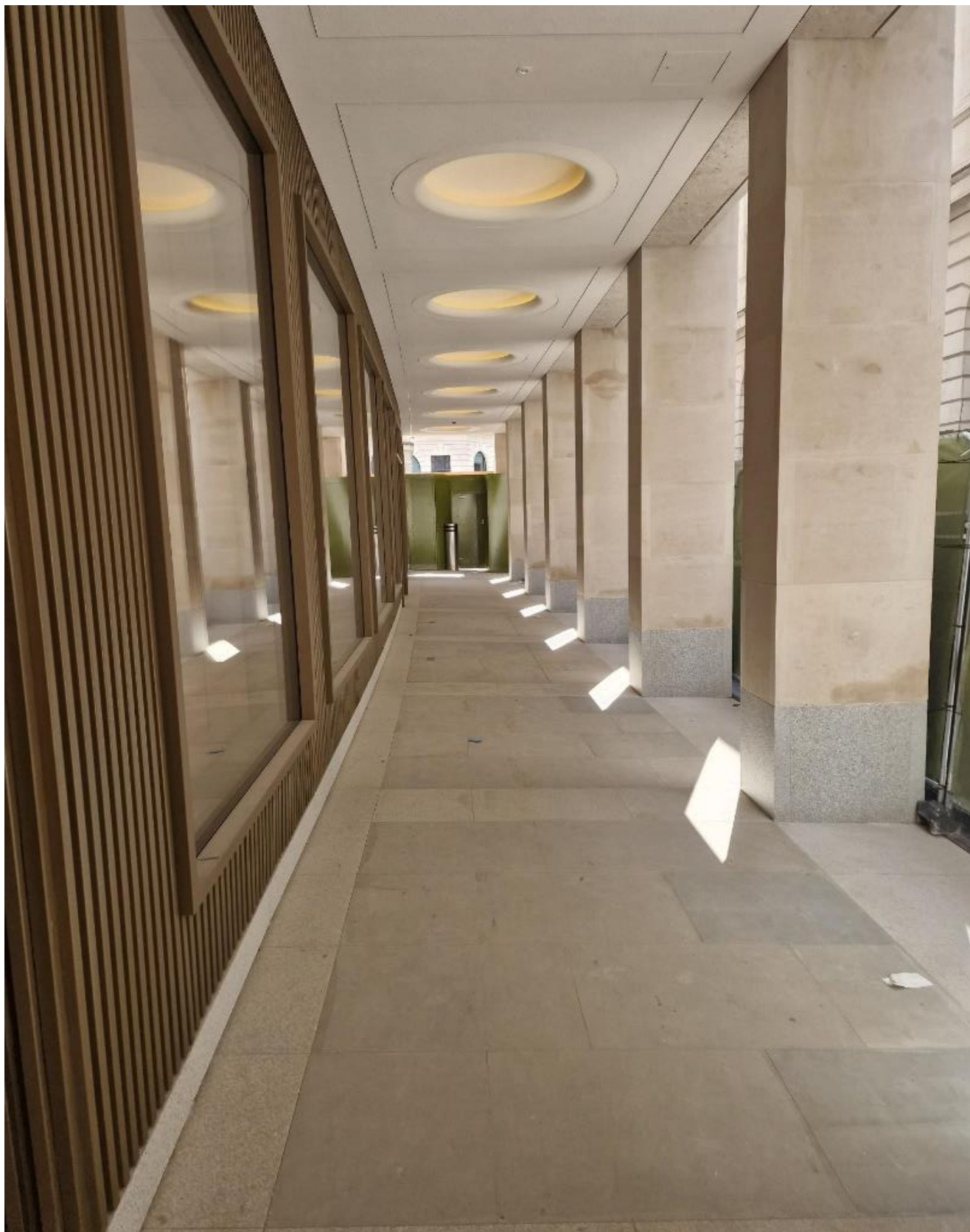
Ironmonger Lane | Dauntsey House Colonnade, recently completed
